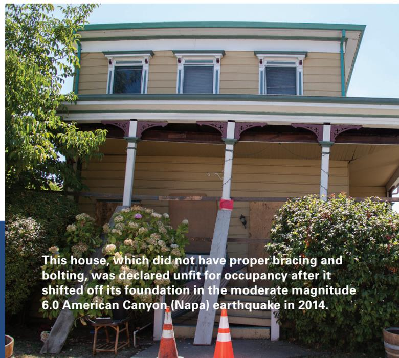
This house, which did not have proper bracing and bolting, was declared unfit for occupancy after it shifted off its foundation in the moderate magnitude 6.0 American Canyon (Napa) earthquake in 2014.
